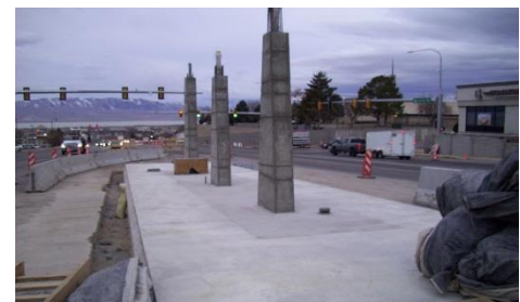
Provo-Orem BRT Platform Construction
